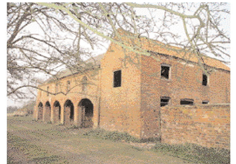
REDUNDANT FARM BUILDINGS, LINCOLNSHIRE © Wanda Sooby
